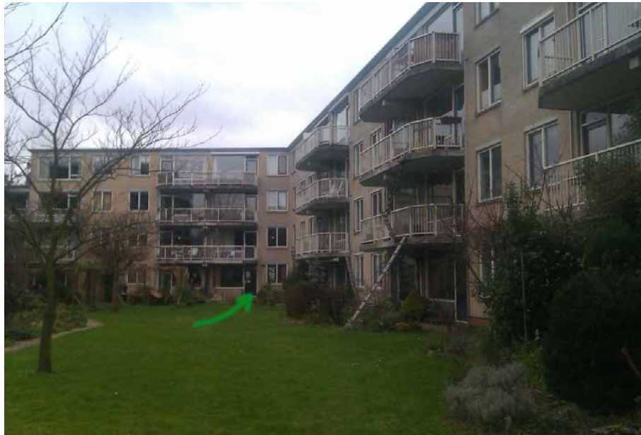
FIGURE 8.4 CW Romolenpolder, common garden with access to common apartment (Tussen Ruimte, 2012)
